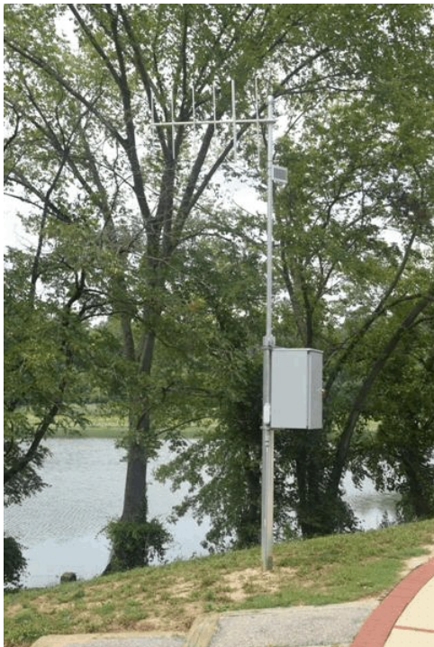
PRGE County Admin Bldg Upper Marlboro
